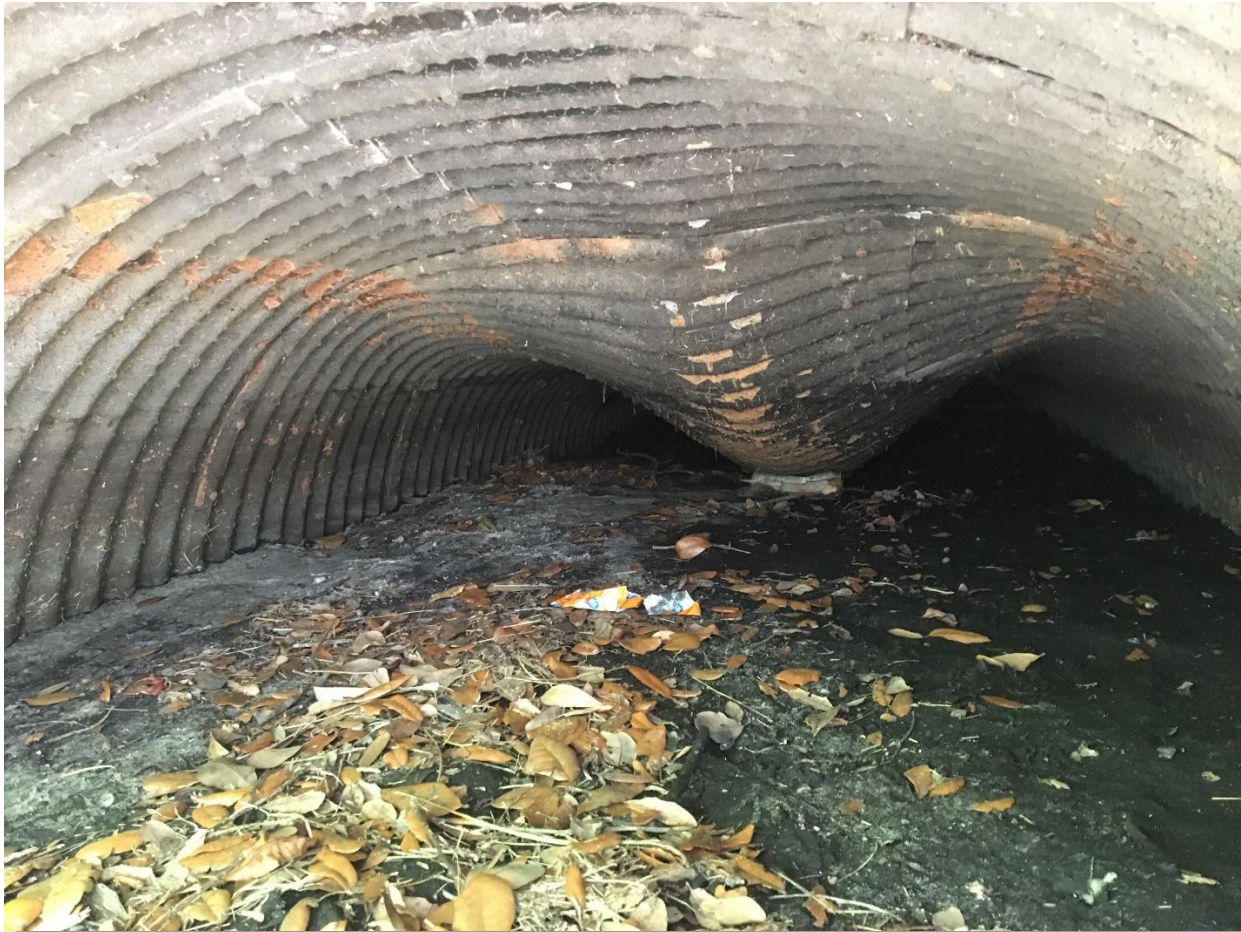
Figure 3 Crushed 48" Storm Pipe, Indiantown, 2019
