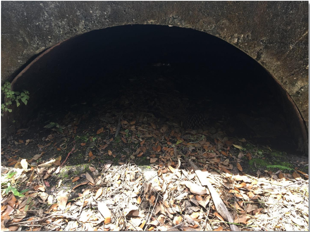
Figure 4 Unmaintained 48" Storm Pipe, Indiantown, 2019
